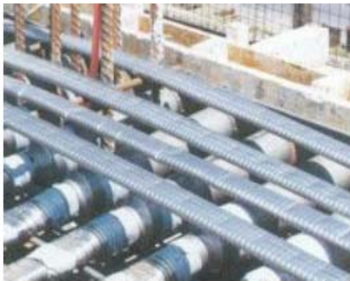
Figure 2.31: Steel flat ducts
