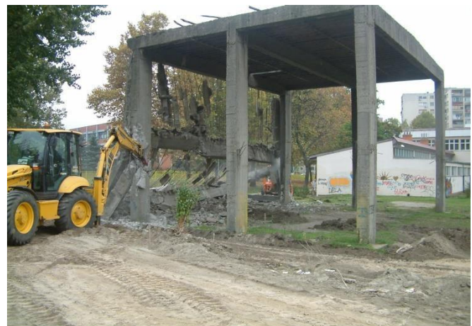
Demolition of concrete structures
